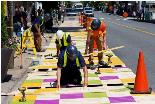
Parklet and bus stop pilot project on Spring Garden Road that was built by HRM. This pilot informed and led to planned investments for permanent streetscape improvements on Spring Garden Road. (Photos by Tristan Cleveland and TJ Maguire)
